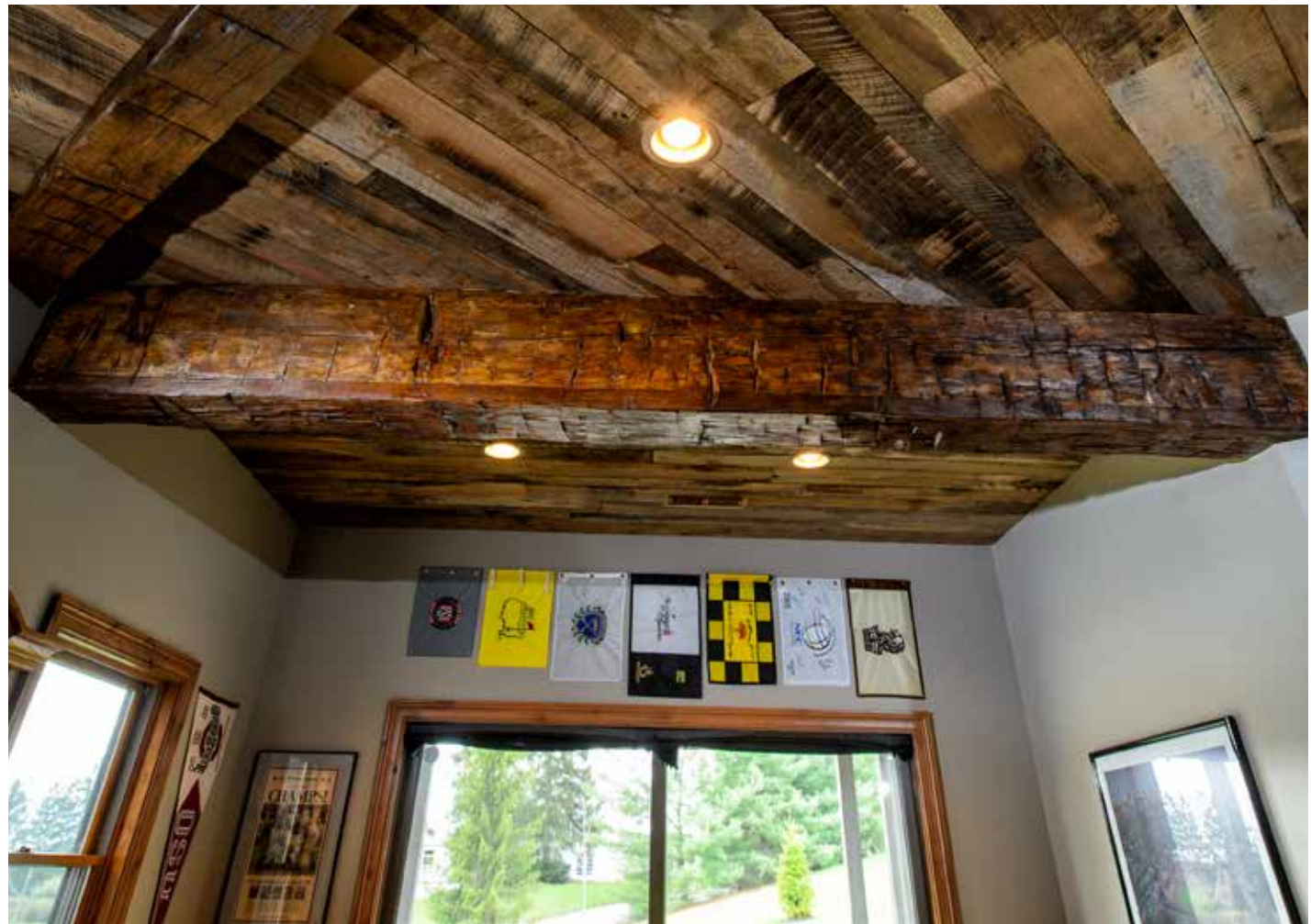
4-SIDED HAND-HEWN BEAM
